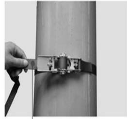
Press the buckle and turn the wrench of the tensioner outwards until the middle buckle falls into the slot. At this time, the lifter can be removed.
