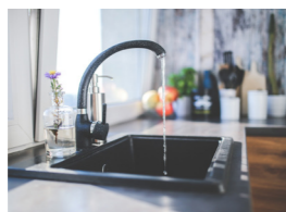
Secondary water supply
